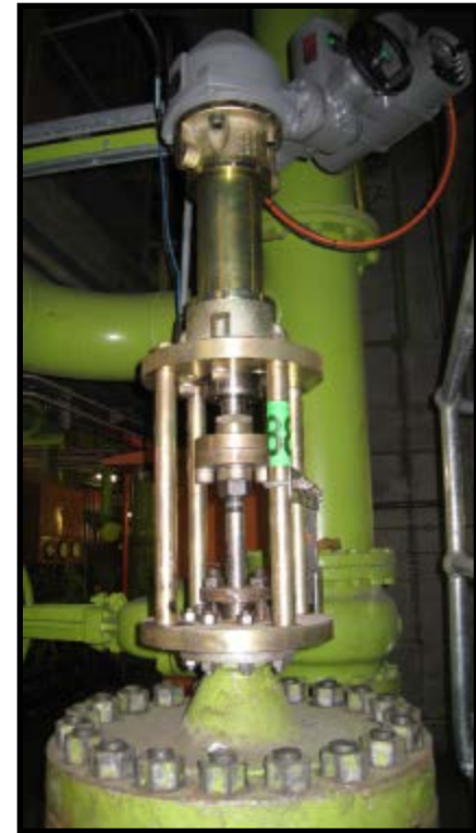
Multi-turn gearbox with linear thrust unit for plug valves (source: AUMA)
