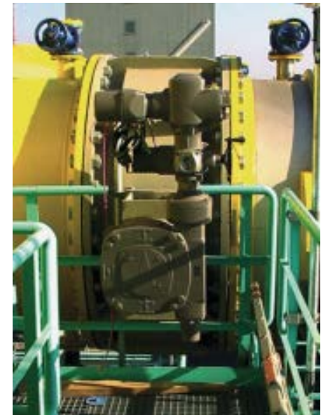
1/4 turn gearbox for butterfly valve automation
