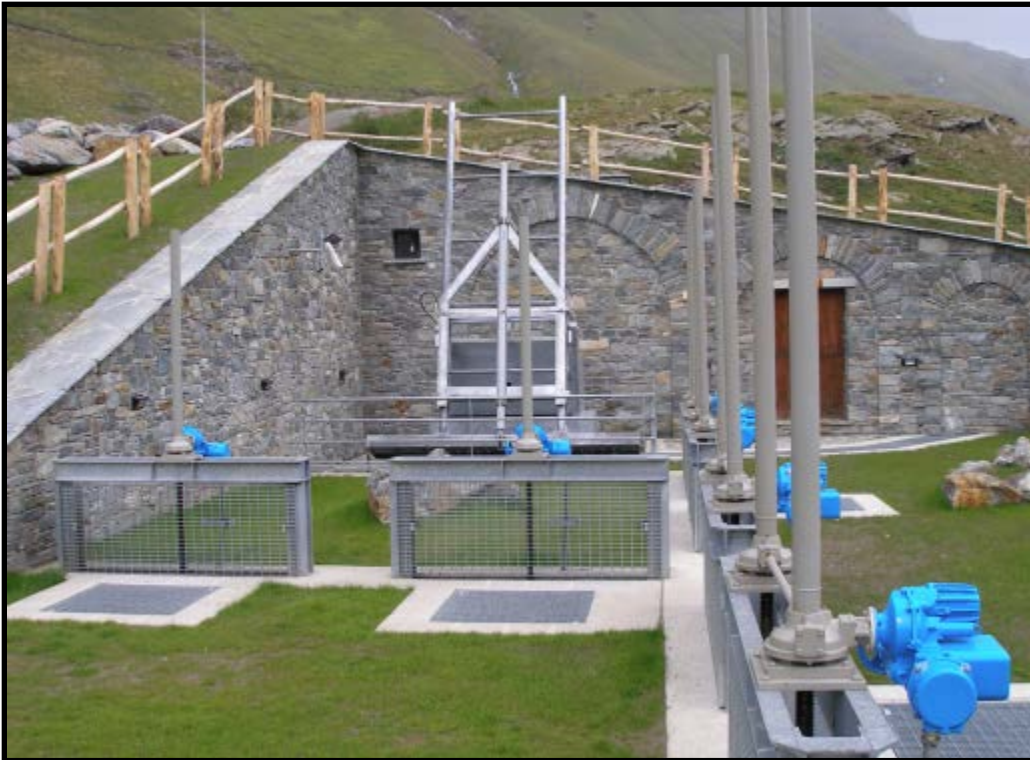
1/4 turn combined with a multi-turn gearboxes for weirs/locks (Source: CML SRL)
