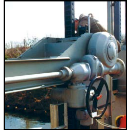
1/4 turn combined with a multi turn gearboxes for weirs/locks (source: AUMA)
