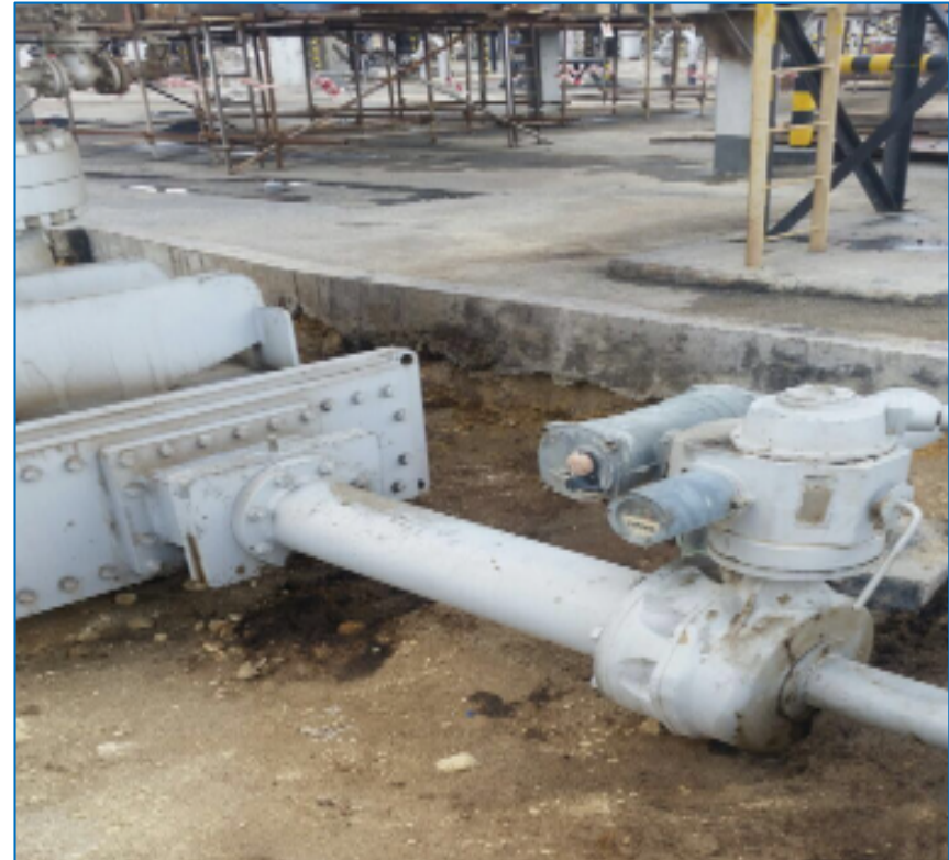
Slab Gate 48" 150 in Crude oil terminal Suffer Stem-Seal leak
