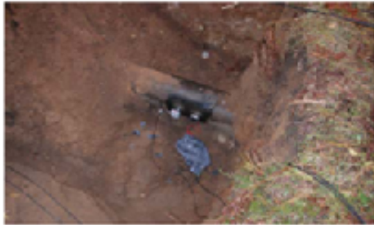
Leak detection in buried pipes
